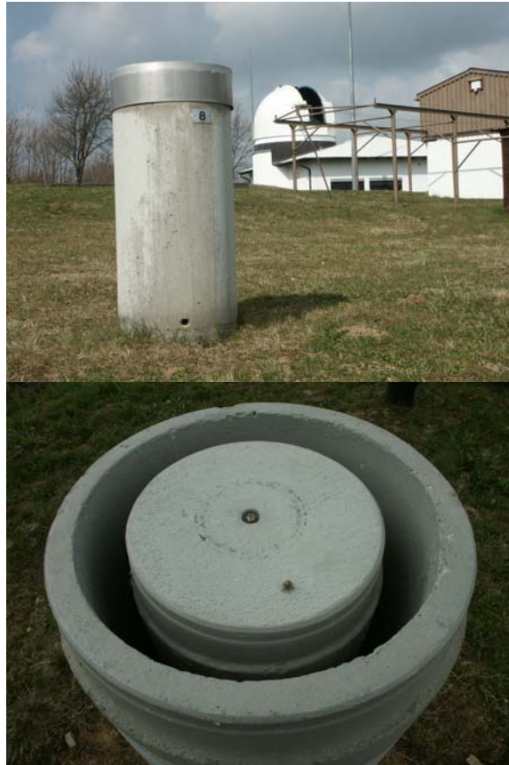
Figure 2: Survey pillar of the local network, top view of the pillar with survey marker for force centering and marker for levelling
